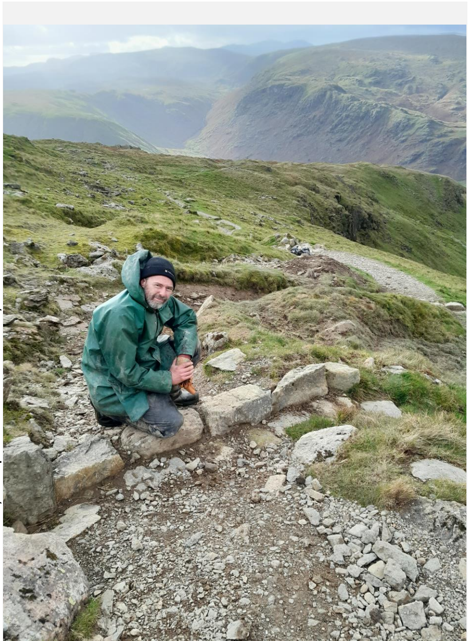
Matt showcases a newly completed water bar at Wythburn
