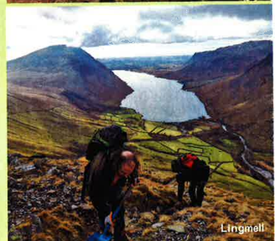
Re-building wall gaps
