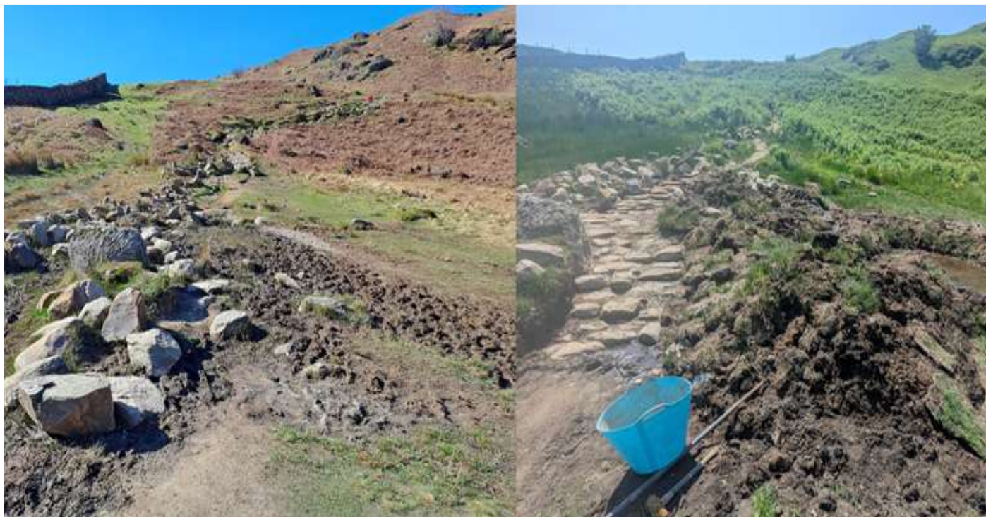
Left: Before: Significant erosion through boggy habitat. Right: After – pitching and wath installed and ongoing pond work.
