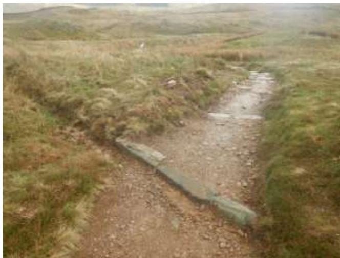
Wansfell path before and after; more steps installed, path widened, drain installed at top to stop water running down path and side route landscaped out.
