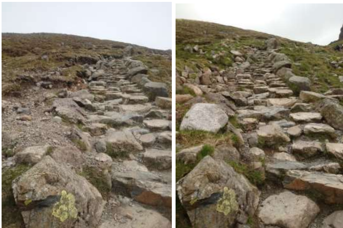
Brown Tongue path up to Scafell Pike at the head of Wasdale, before (left) and after (right) work by the team to repair erosion damage
