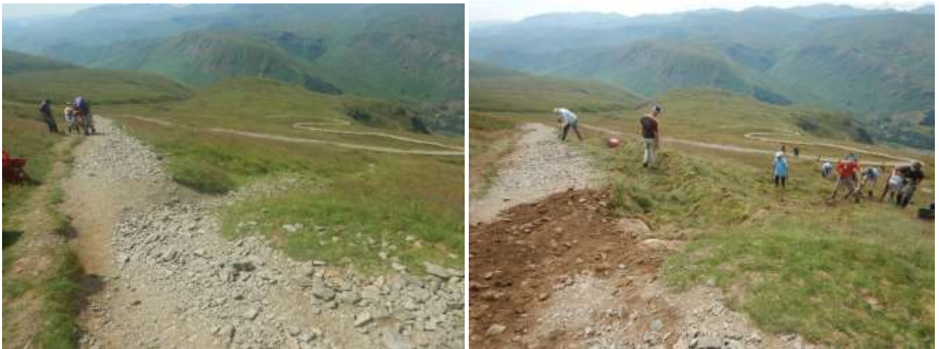
A shortcut on the path up to Helvellyn from Wythburn – before work (left) and during landscaping work by volunteers to hide the eroding line and encourage people to stay on the path (right).
