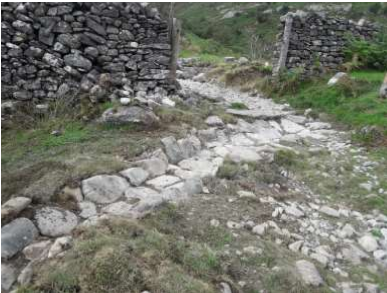
Rebuilding the Borrowdale megadrain on the Rigghead Quarries path!
