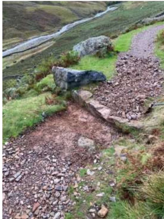
The upland path on Bursting Knott Wasdale (left) – spot the drain? There is one here! After much shovelling and sweeping, as if by magic, a drain appears (right).
