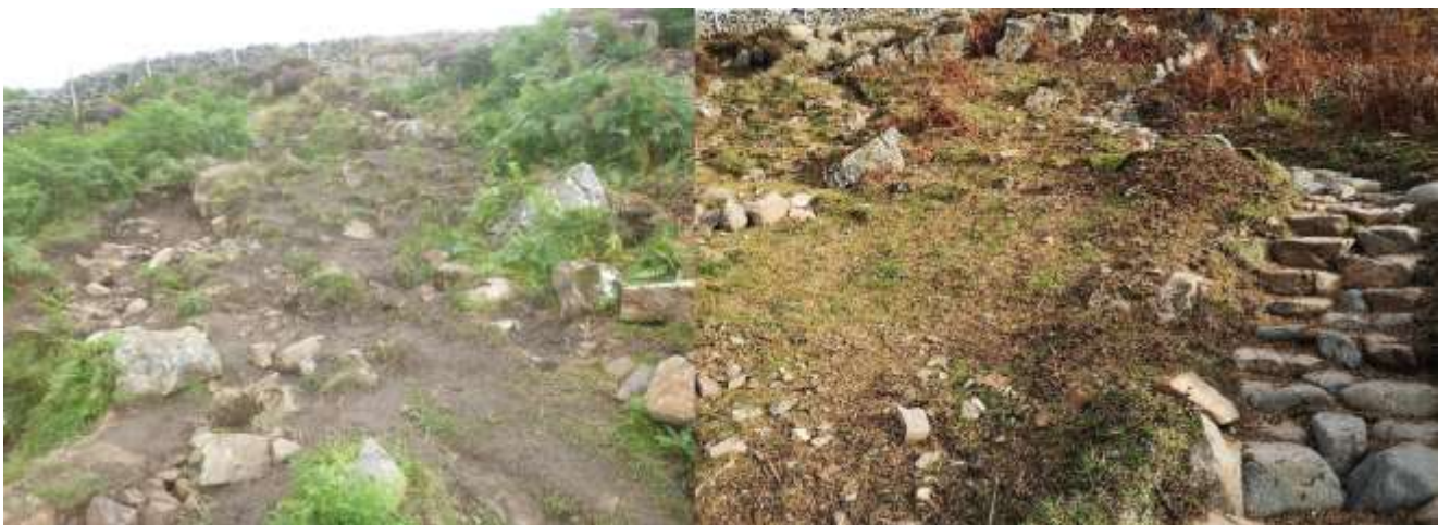
Gowbarrow before (left) and after (right) landscaping and installing new pitching
