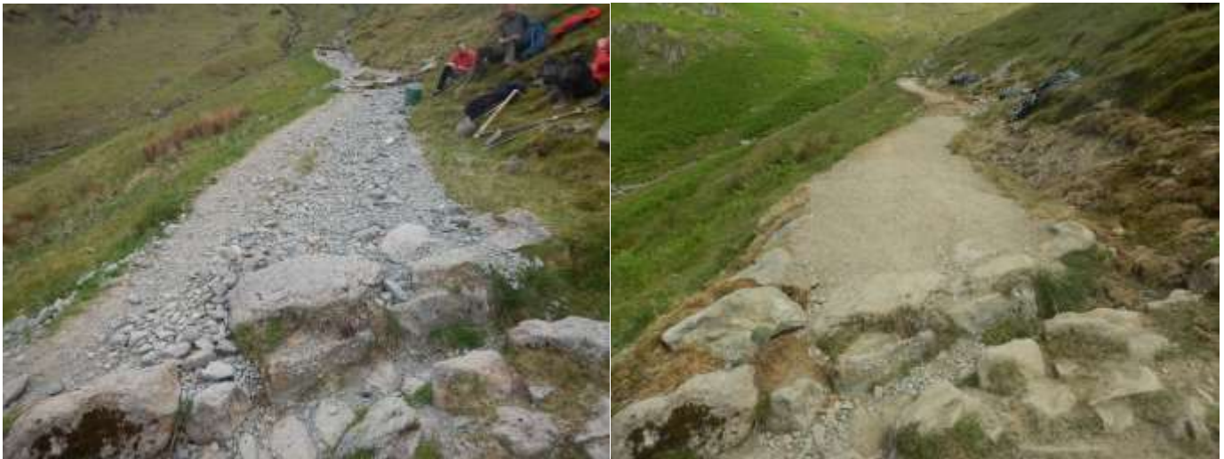
Wythburn path before (left) and after (right) constructing a "roman" style path
