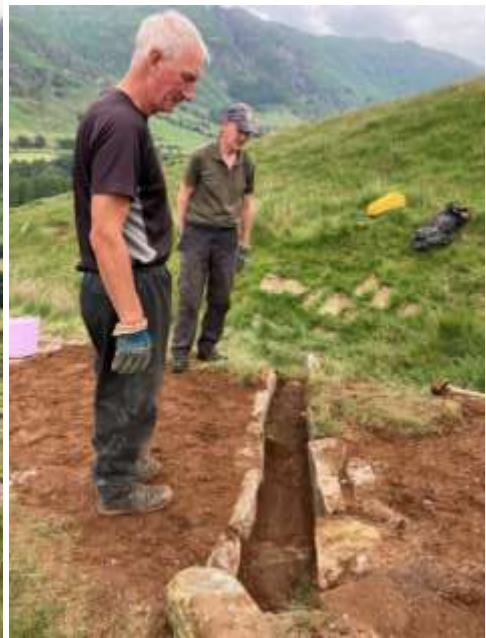
Left - Volunteers Alan and Richard start building a new drain on Side Pike, Langdale (left) and the finished product (right)
