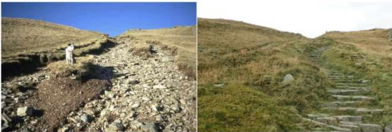
Garburn to Yoke – Before (2001) and after (2019) work by Fix the Fells
