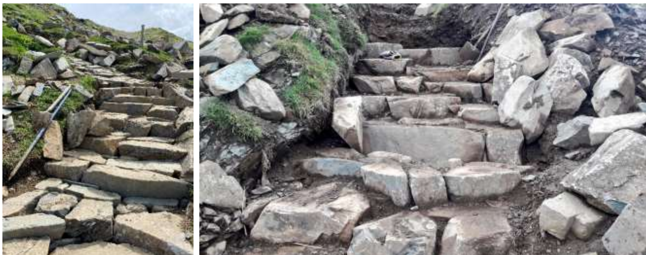
Left - Section of new pitching which has replaced some old sloped stone work. Right - Stone risers through a gully.
