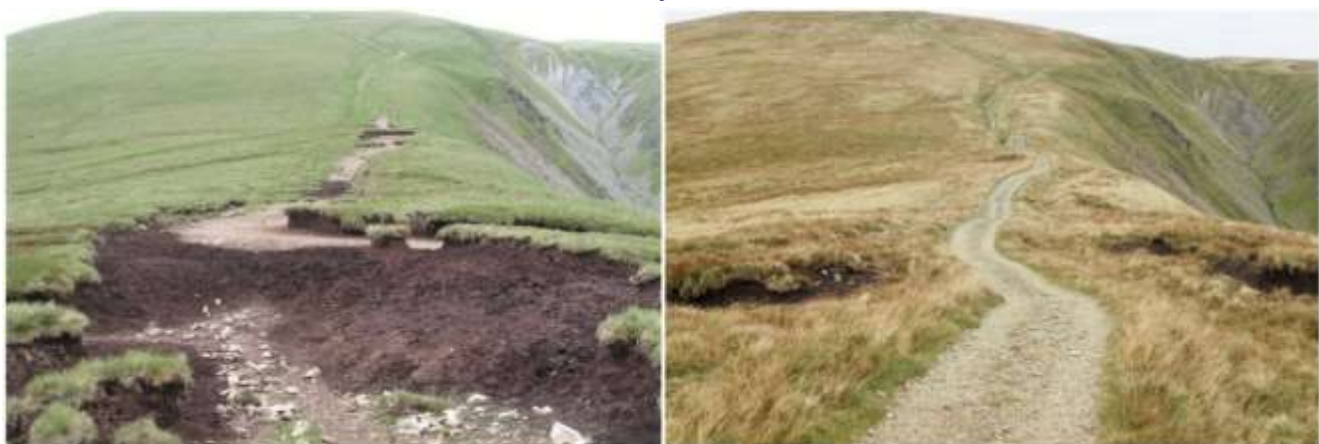
Thornthwaite Beacon, Kentmere - Before (2005) and After (2019) work by Fix the Fells
