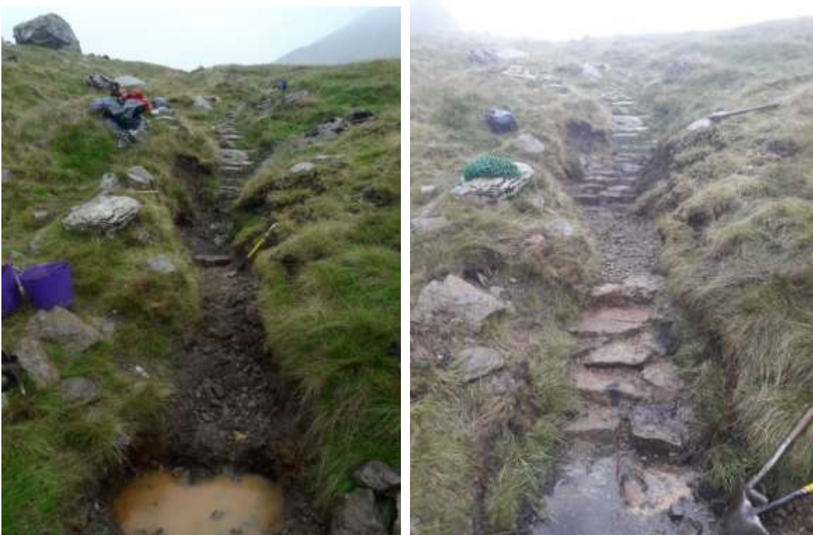
Repairing a badly gullied section of the Coast to Coast at Tongue Ghyll, Grasmere – during (left) and after work (right)
