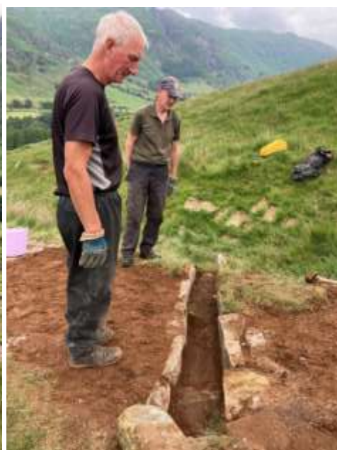
Volunteers Alan and Richard start building a new drain on Side Pike, Langdale (left) and the finished product (right)
