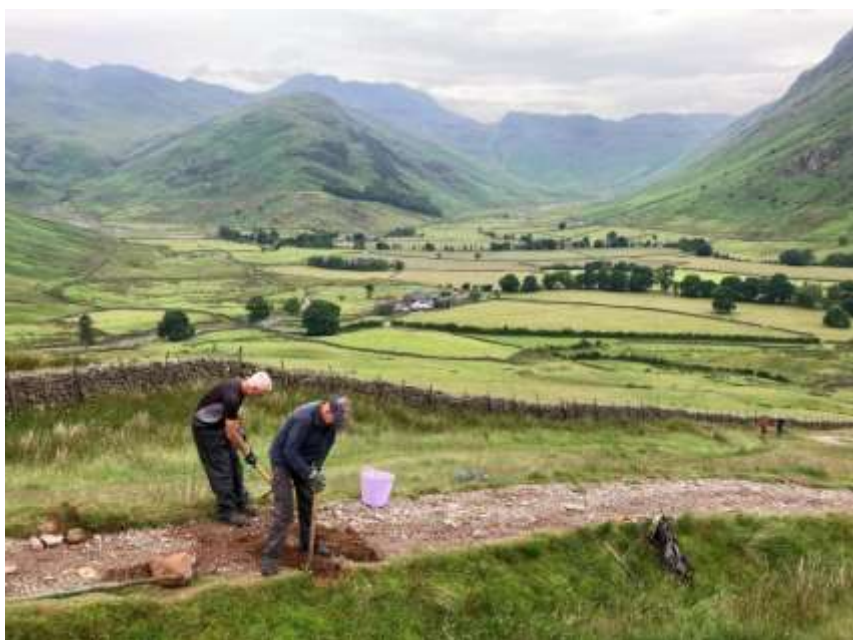
Volunteers Alan and Richard start building a new drain on Side Pike, Langdale (left) and the finished product (right)
