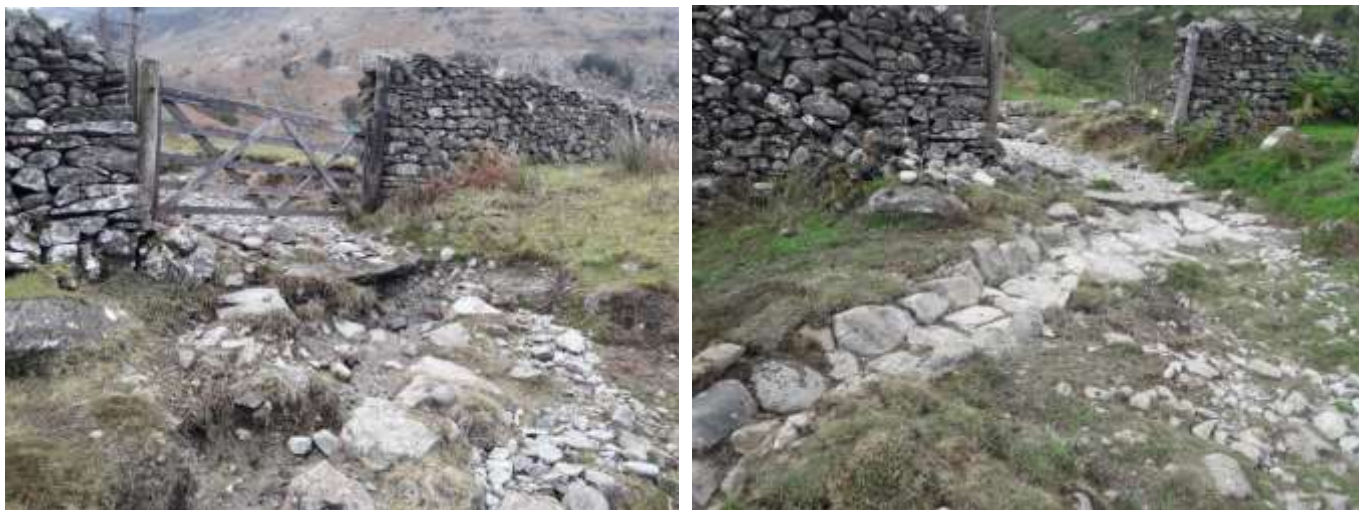
Rebuilding the Borrowdale megadrain on the Rigghead Quarries path!
