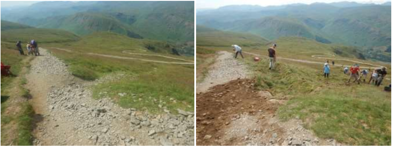
A shortcut on the path up to Helvellyn from Wythburn – before work (left) and during landscaping work by volunteers to hide the eroding line and encourage people to stay on the path (right).
