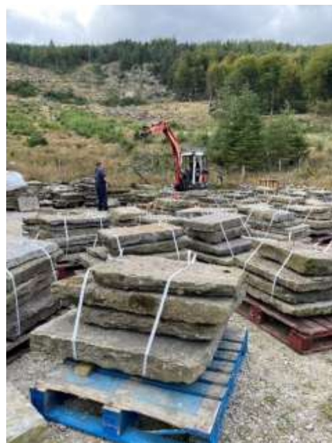
Coast to Coast path over Greenup Edge (left) and stone flags ready to be flown by helicopte to create a path (right)
