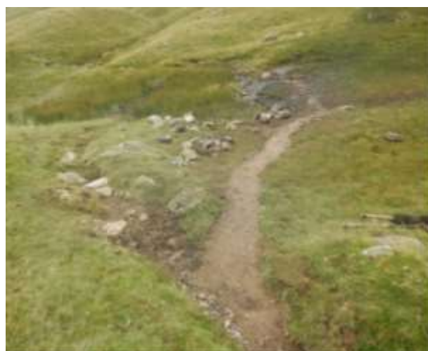
Langdale Coombe: Left picture – old path leading to bog, reeds and ground to the right trampled by walkers seeking drier line. Right picture – old path closed, new line and ‘high and dry’ causeway installed
