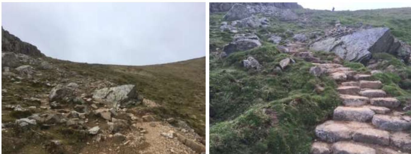
The path on Calf Cove before (left) and after (right) work
