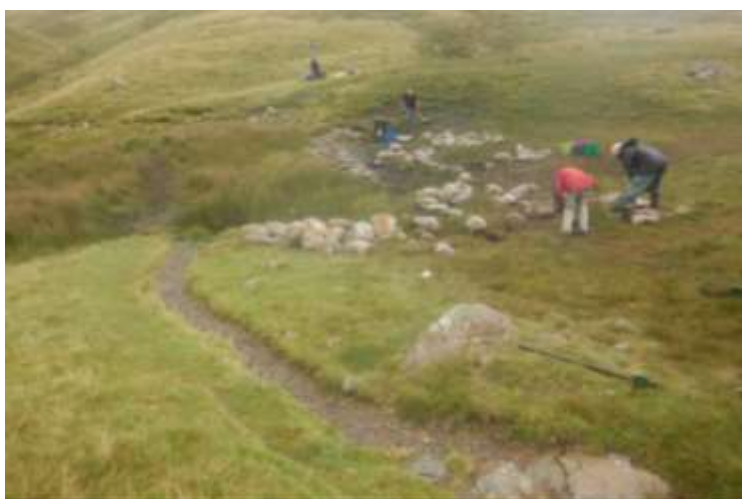
Langdale Coombe: Left picture – old path leading to bog, reeds and ground to the right trampled by walkers seeking drier line. Right picture – old path closed, new line and ‘high and dry’ causeway installed
