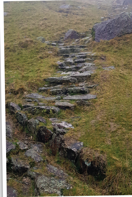
A typical section of the pitched path, with a cross-drain in the foreground
