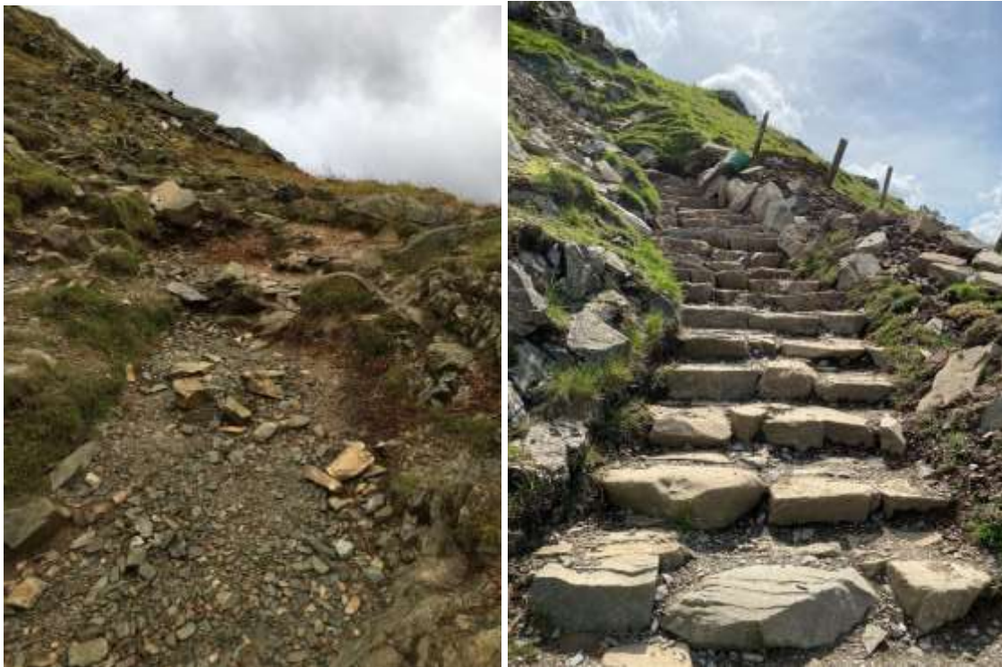
Badly eroded ground (left) and new sustainable stone path (right) on Loughrigg Fell above Grasmere.
