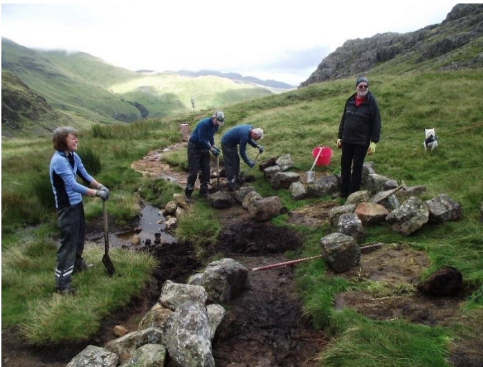
Left: One of our unsupervised work parties extending pitching on the top of the Browney Gill path in Langdale.
